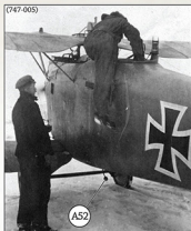
A crew member climbs into early production Hannover CL.II 9224/17 during the winter of 1917-18. Note the small flares and flare gun, partially hidden by his right leg. There is an additional gravity tank fixed above the top wing.
